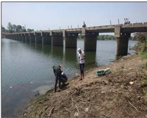
Picture: River Betwa, near Road Bridge, Ganj Basoda
