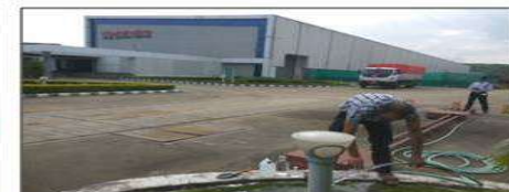
Picture: Ground water Monitoring : M/S, Mahindra Steel Service Centre, Mandideep
